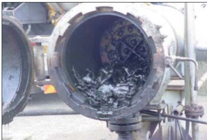
Pre-cleaning of Total's 140-km crude transport line to its refinery in Vlissingen, the Netherlands, removed the wax and paraffin shown here in a trap at the refinery (Fig. 1).
