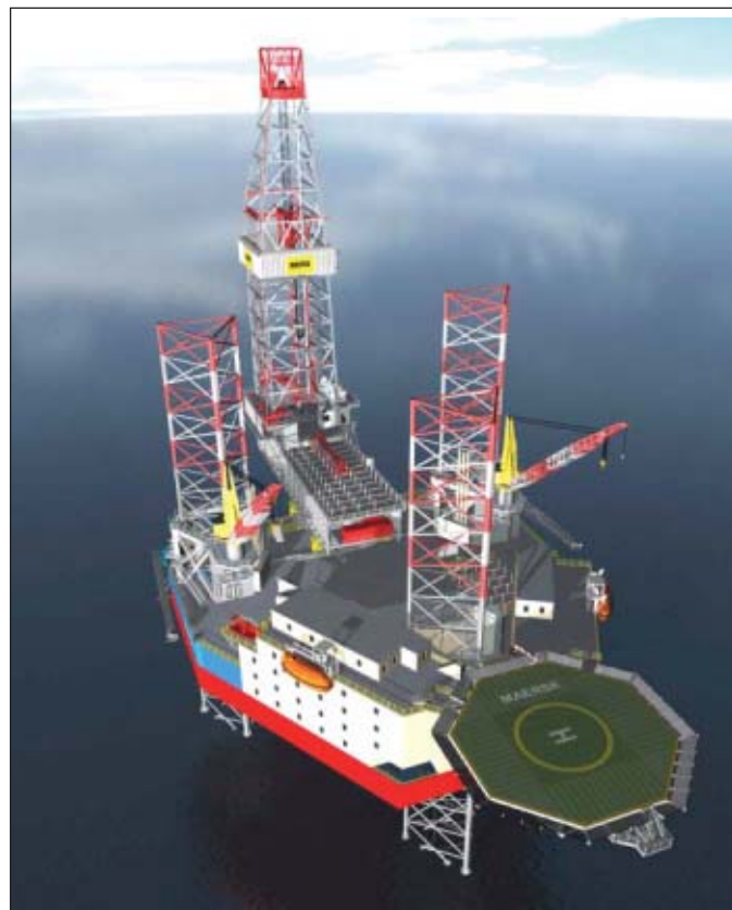
Marine Structural Consultants BV and Maersk designed the new 350-ft CJ-0-X100 MC cantilevered jack up (Fig. 2, image from Maersk).
