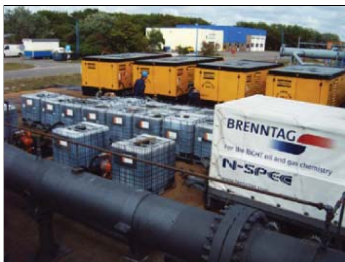
Brenntag used this 24-in. pig launcher at the Maasvlakte Oil Terminal to launch the four-pig train used to clean Total's crude transport line. This picture also shows the chemical units that injected dispersant and cleaning agents between the pigs and the compressor units used to push the train towards the refinery with compressed air (Fig. 3).
